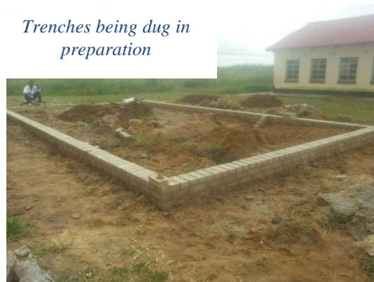
Foundations for the kitchens
