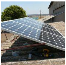
Solar panels fitted on site in Zimbabwe
