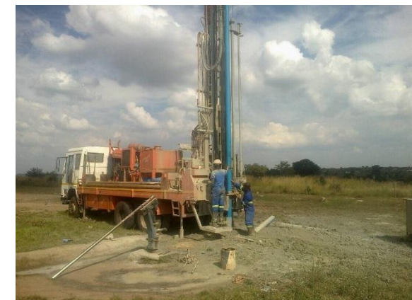
Bore hole installation
