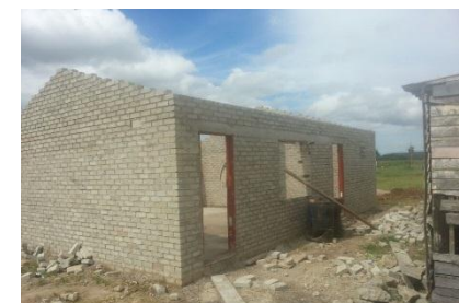
Kitchens reaching completion
