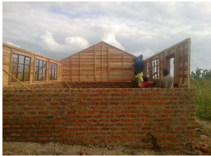
Classrooms being built in MB
